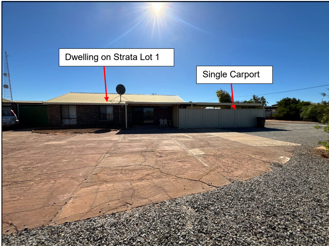
View of 1a Mead Street from the west / driveway side
