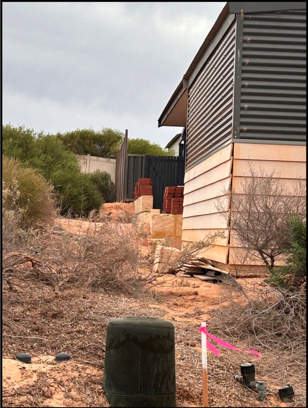
Above: View of development to the north at 29 Freycinet Drive
