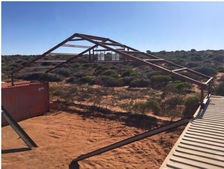
PHOTOGRAPH OF ROOF FRAME ATTACHED TO 2 SEA CONTAINERS
