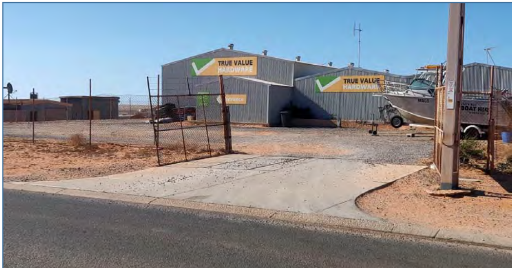
Right hand side unconstructed crossover
