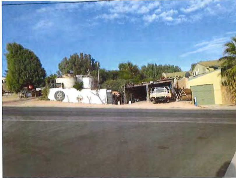
Photo of Lot 100 Durlacher Street showing existing structure
