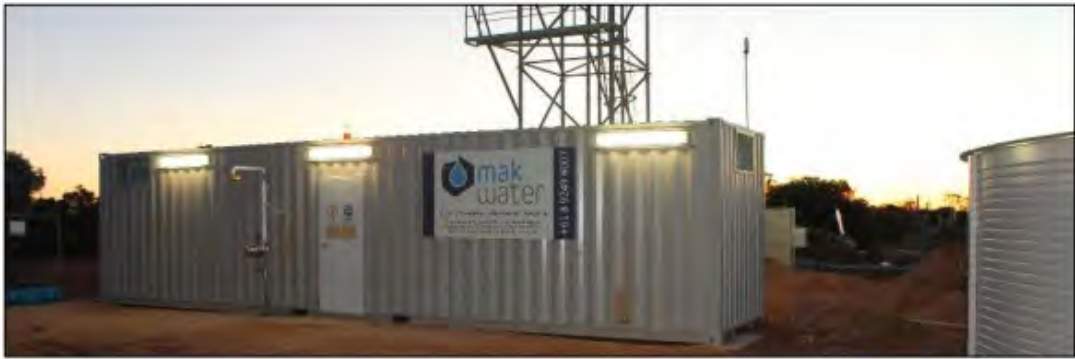
A MAK Water containerised RO plant with ClearAccess™ installed on a remote site
